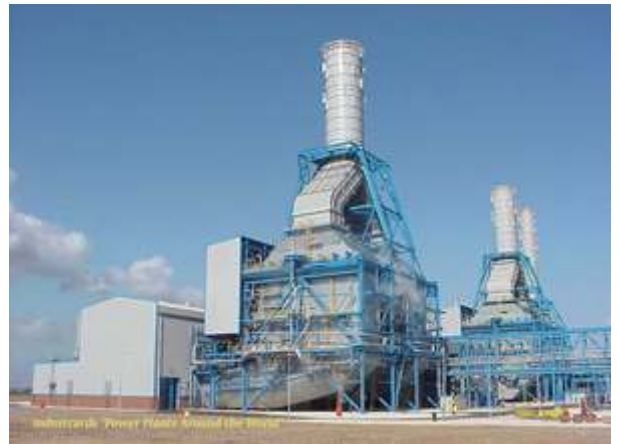
South Humber Bank Power Station
