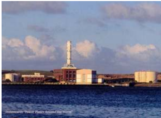
Roosecote Power Station
