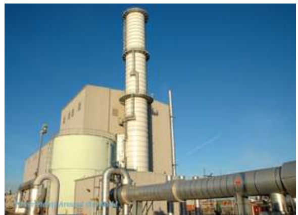
Great Yarmouth Power Station
